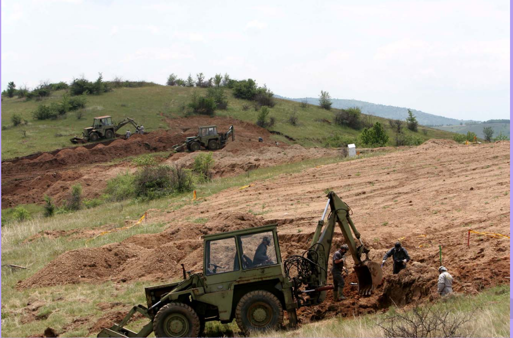
Borovac, southern Serbia, 2007. Earth moving equipment is used to reveal buried penetrators.
